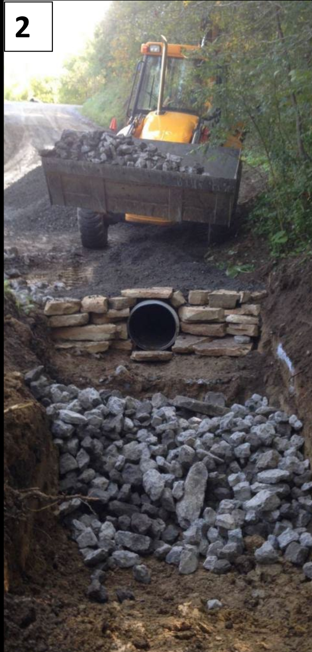
3' Deep, filled w/ R4 and edged with pallet stone.
