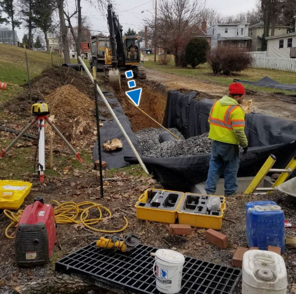
Dauphin, 31 st St 6/8 • Installed drop inlets to “cascading” subsurface infiltration structures
