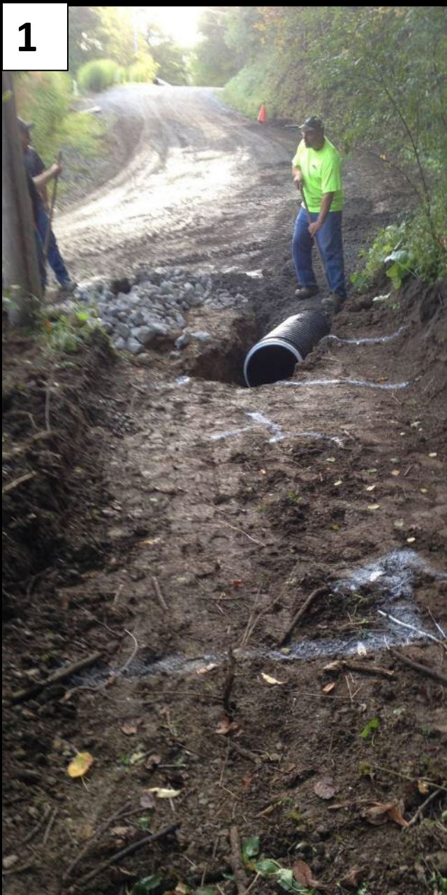
3' Deep, filled w/ R4 and edged with pallet stone.
