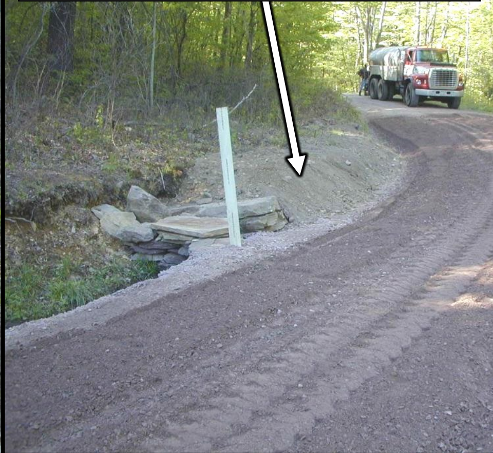
After: Imported bank material
