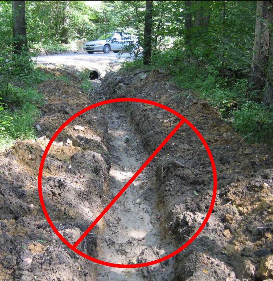
Cover obtained by digging
