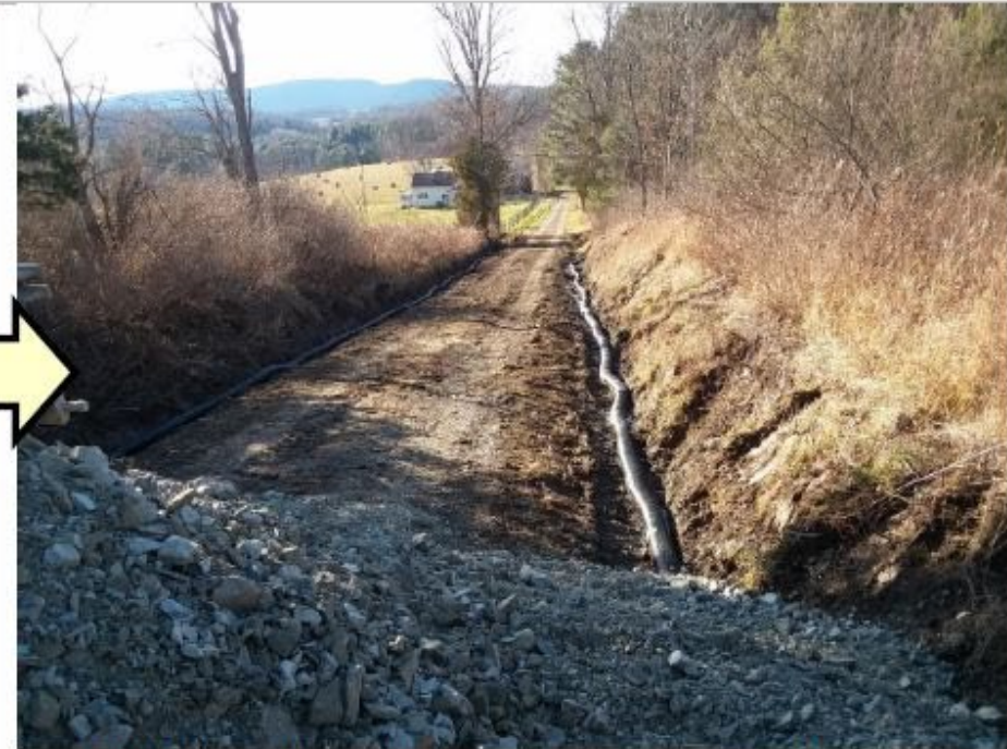
DURING: Fill provided needed cover for under drain
