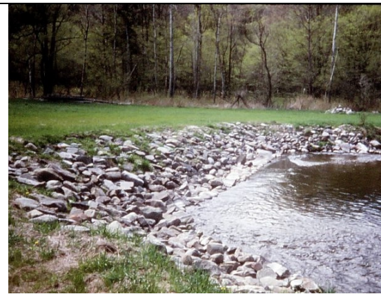
Butternut Creek After Stabilization
