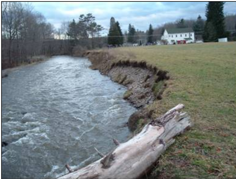
Nonpoint source problem area #52 Streambank is in need of restoration
