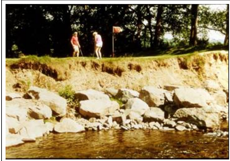
Streambank erosion problem area along Wallenpaupack Creek before restoration
