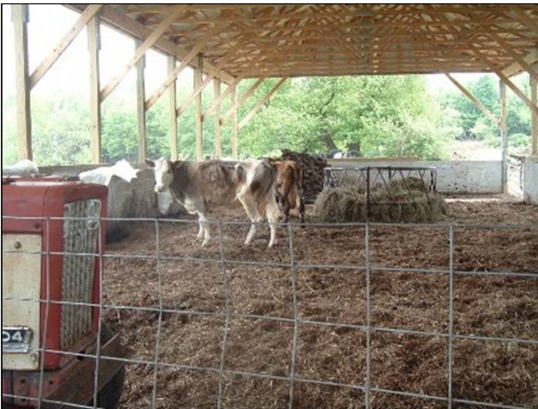
Inside of Agricultural Waste Facility After BMP Construction
